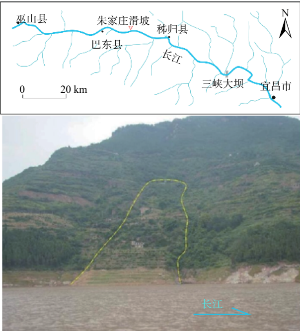
图 6 朱家店滑坡全貌 [20] Fig. 6 Overall perspective of the Zhujiadian landslide
