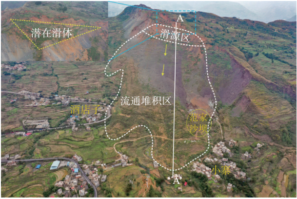
图 2 尖山营滑坡碎屑流全貌 Fig. 2 Overview of Jianshanying landslide-debris flow
