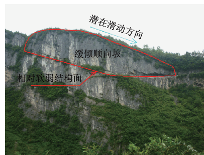
图 5 武隆天生三桥缓倾顺向边坡照片 Fig.5 The photograph of gently slant slope in Wulong Tiansheng bridge
