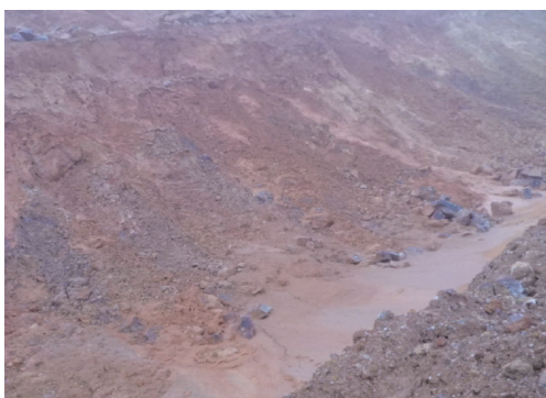
图6 持续降雨诱发的水土流失 Fig. 6 Soil erosion induced by sustained rainfall
