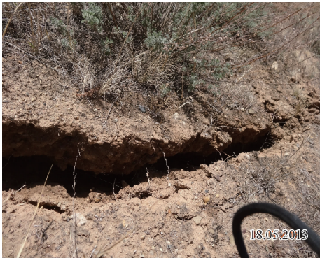
图 4 滑坡后缘处的张拉裂缝 Fig.4 The tensile cracks at the edge of the landslide
