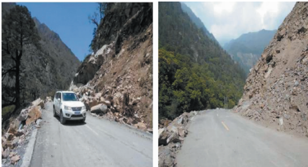
图 2 G216 沿线崩塌灾害 Fig.2 Collapse disaster along G216
