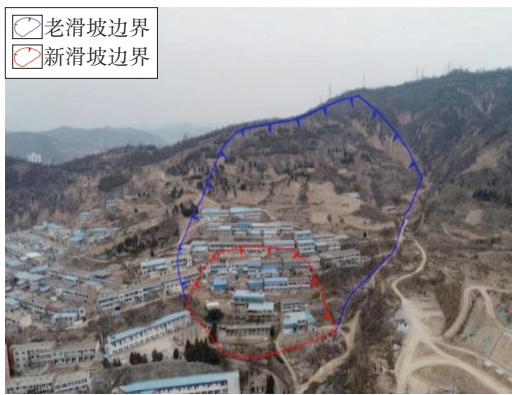
图 1 二庄科滑坡全貌 Fig. 1 Overview of the Erzhuangke landslide
