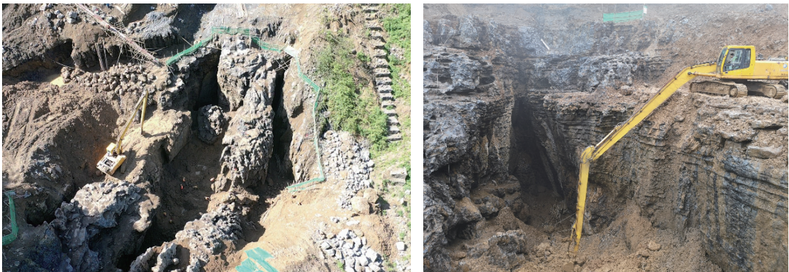
图 4 挡墙基础岩溶开挖图 Fig. 4 Excavation pictures of the karst for foundation of the retaining wall
